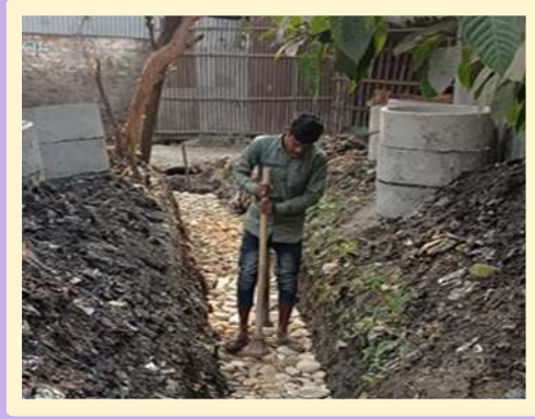
Drain construction at ward no. 45
