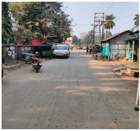
NAME OF WORK : Upgradation of Colipara main road Hill Cart Road to 4th Mahananda setu under Siliguri MC ESTIMATED AMOUNT : Rs. 63,09,609
