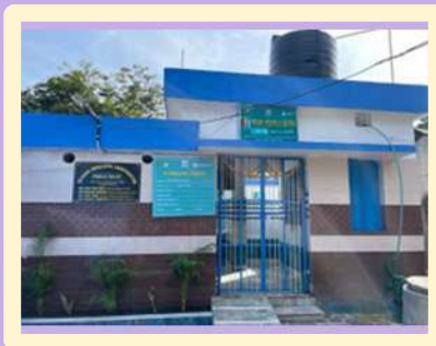
Inauguration of Community Toilet at Rana Basti Ward no. 18
