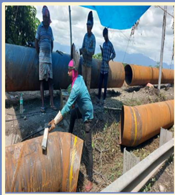
LAYING OF PIPELINE
