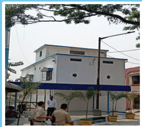
NAME OF WORK : Repairing and upgradation of APC Sarani 1 from DBC road to PIPE line under Siliguri MC ESTIMATED AMOUNT : Rs. 62,51,105
