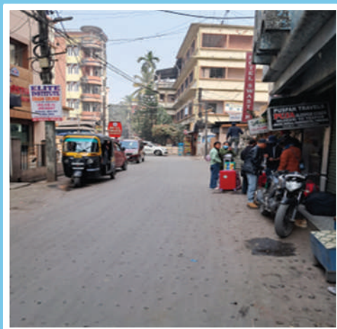
NAME OF WORK : Repairing and upgradation of road Beside Delhi hotel to Nivedita road and to Gurung basti main road under Siliguri MC ESTIMATED AMOUNT : Rs. 40,12,808
