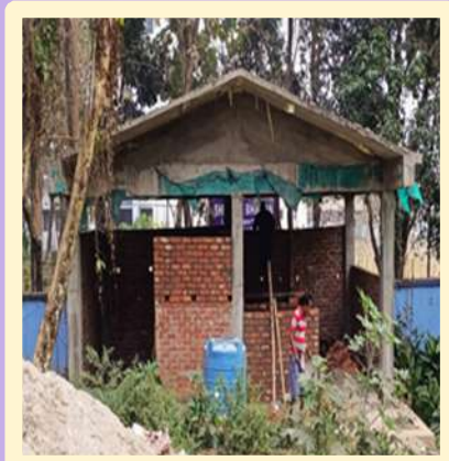
Public Toilet Construction at Ward no. 46
