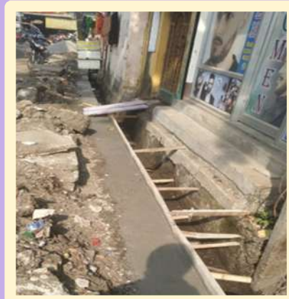
Drain construction at ward no. 37
